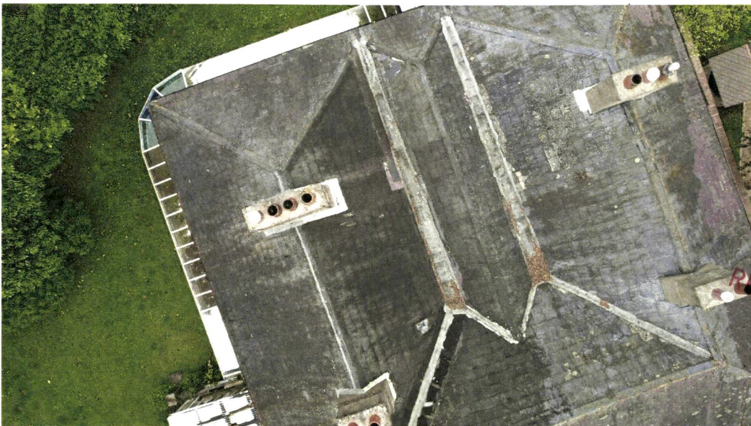
Aerial shot of the whole roof showing the structure
