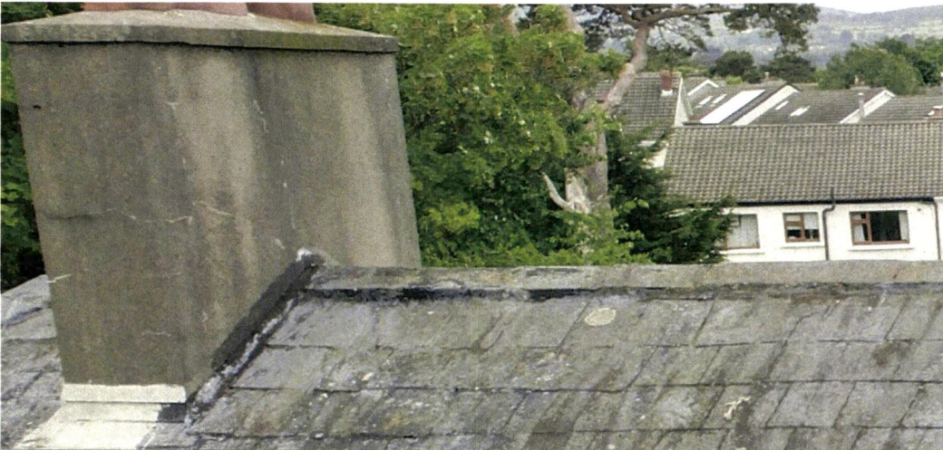
Flashing repairs around the chimney,
